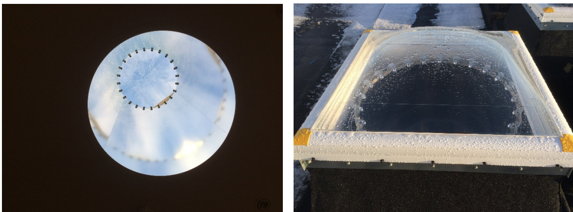
Figure 31 Shopping centre, Trondheim, Norway. The artificial lighting system based on LED was integrated on the top of the light tube. Left: light tube from inside; right: light tube from outside (Pictures: SINTEF)
